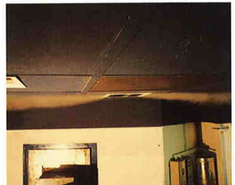
Picture 1 Horizontal two-way throw at 77 CMH
