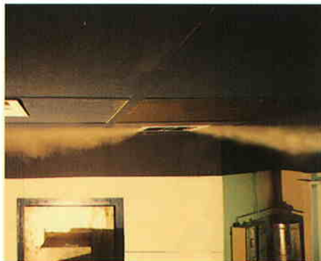
Picture 2 Horizontal two-way throw at 204 CMH
