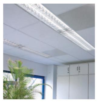
Figure 6: Opticlean installed in a grid ceiling
