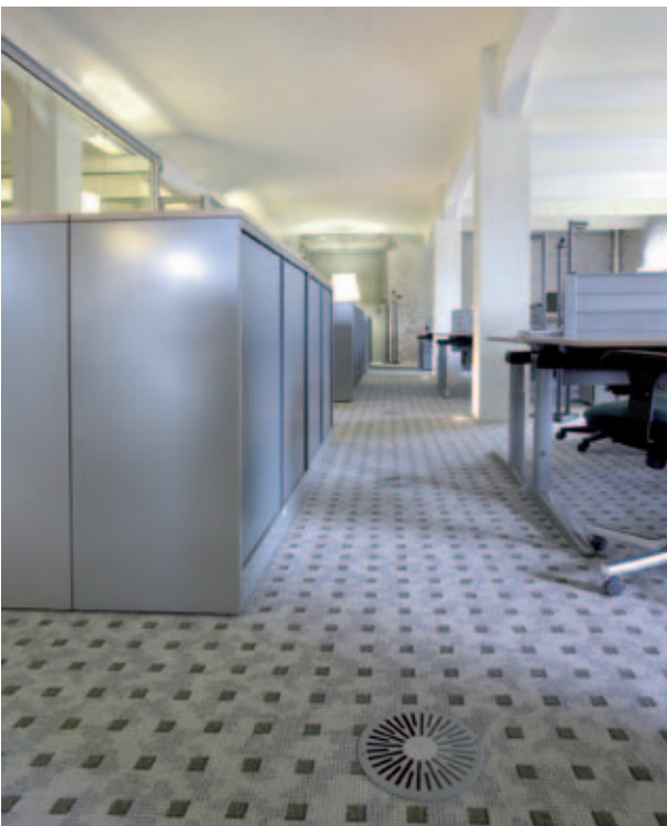
Figure 6: Floor twist outlet in an office
