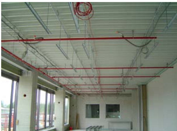
Fig. 7: For panel suspension, the fastening crossbars are suspended from the ceiling using threaded rods and their position is adjusted in height and alignment
