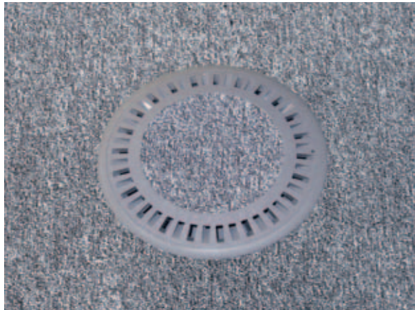
Fig. 2: Floor displacement outlet in a raised floor
