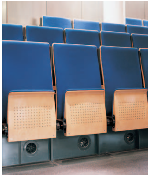
Fig. 5: Step twist outlets DD-DD-DN 100 in a lecture hall
