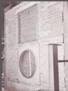
FIG 4B Fire dampers 145 minutes after the start of fire resistance test.
