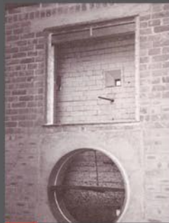
FIG 4A Fire dampers before the fire resistance test.
